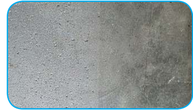
Before and after shotblasting
