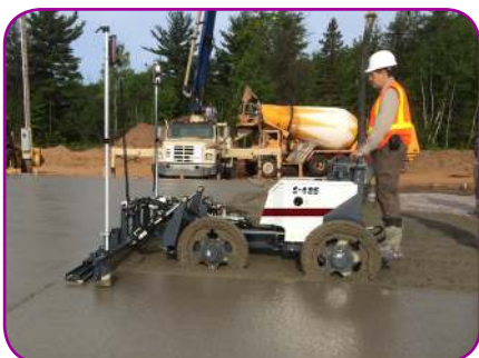
S-485 Laser Screed® equipment on the job
