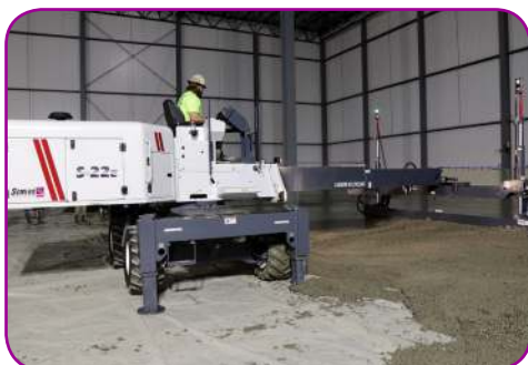
S-22E Laser Screed® equipment on the job
