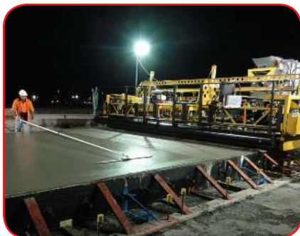
255CD on the job
