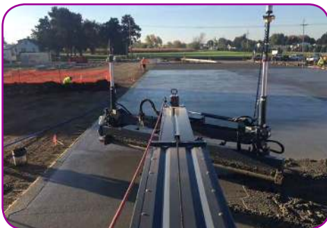
S-22EZ Laser Screed® equipment on the job
