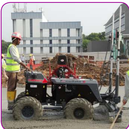
PowerRake® 3.0 on the job
