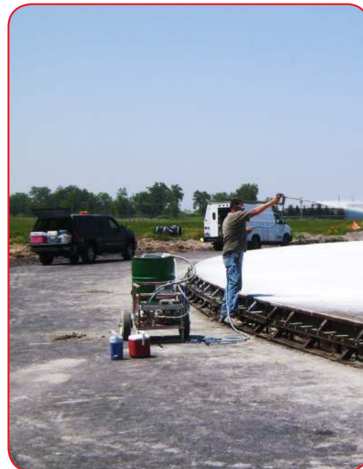
*9910 Power Sprayer on the job
