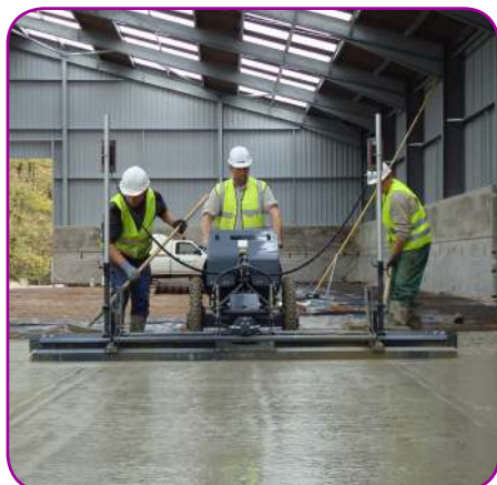
Copperhead XD3.0 Laser Screed® equipment on the job
